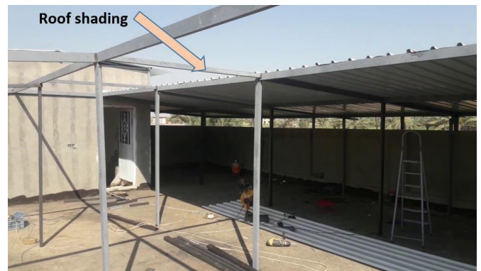
Fig. 1 Roof shading in Iraq.
